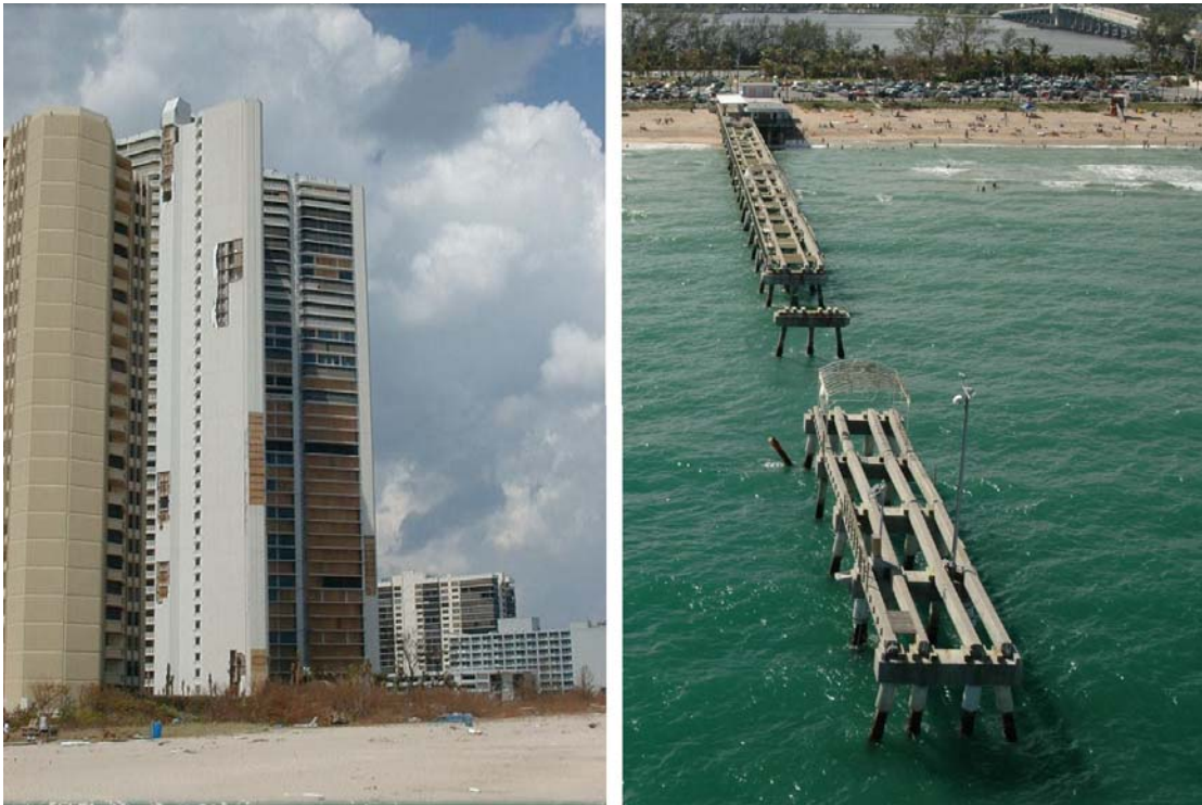
Photo 35: Wind Damage, Riviera Beach (R70) & Damage to Lake Worth Pier
