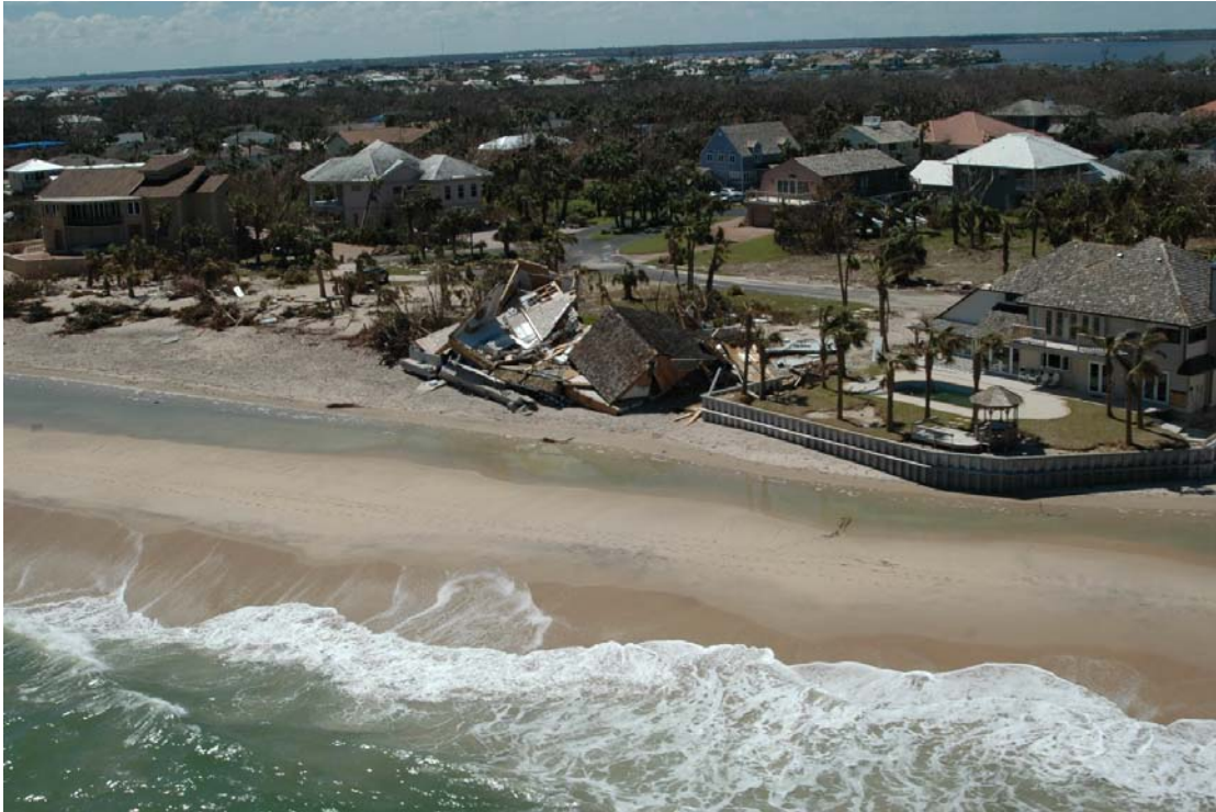
Photo 24: Destroyed Residence, South Vero Beach
