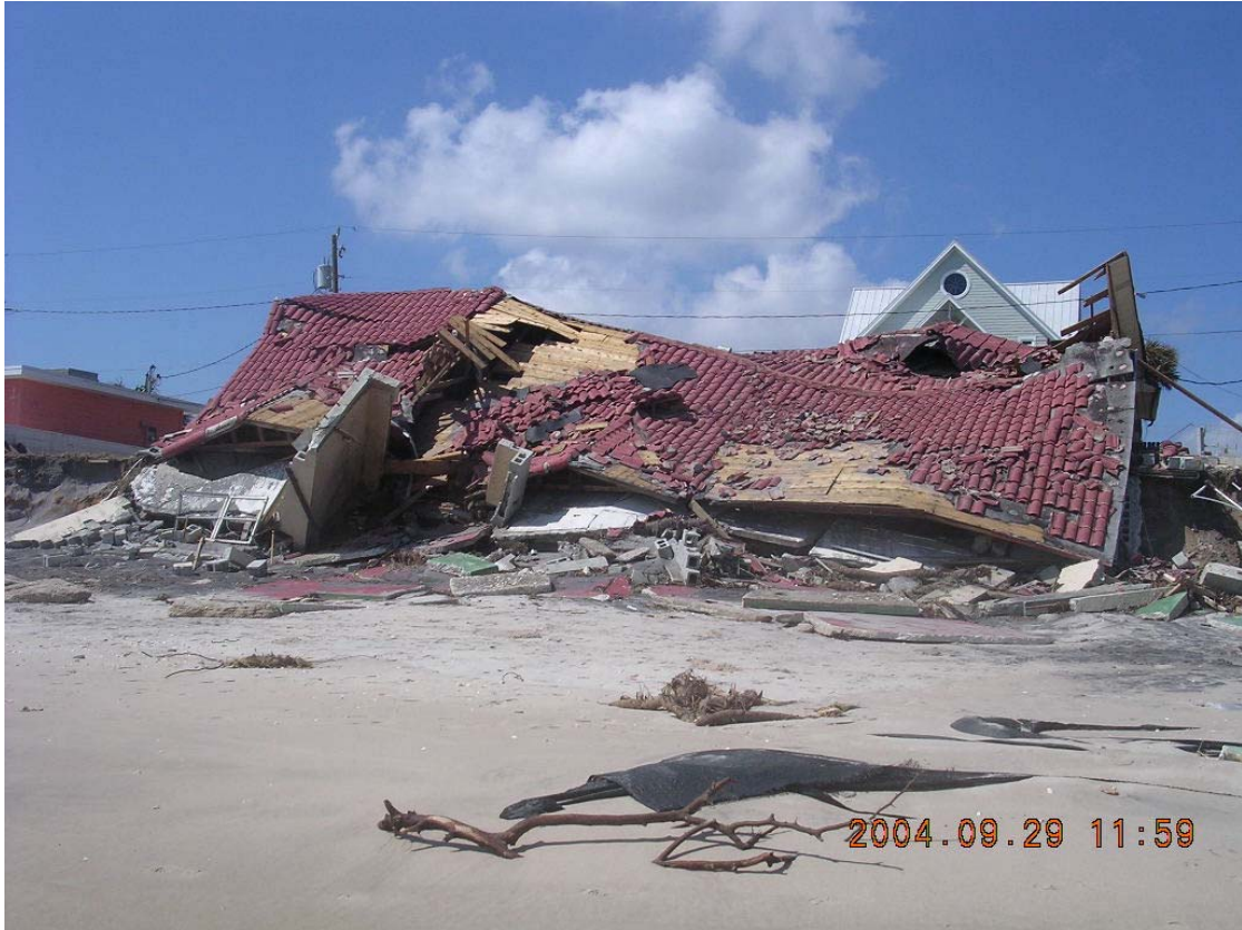
Photo 9: Ocean Lane Residence Destroyed, Satellite Beach
