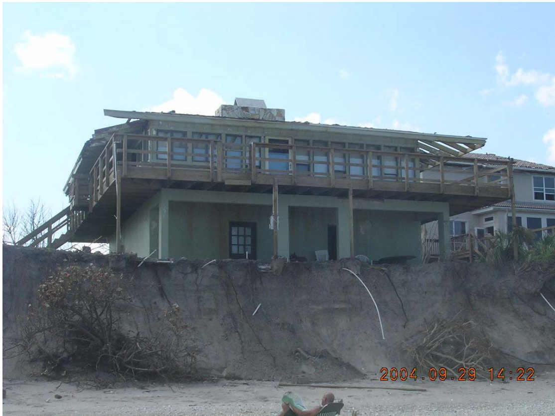
Photo 15: Major Dune Erosion Threatens Residence
