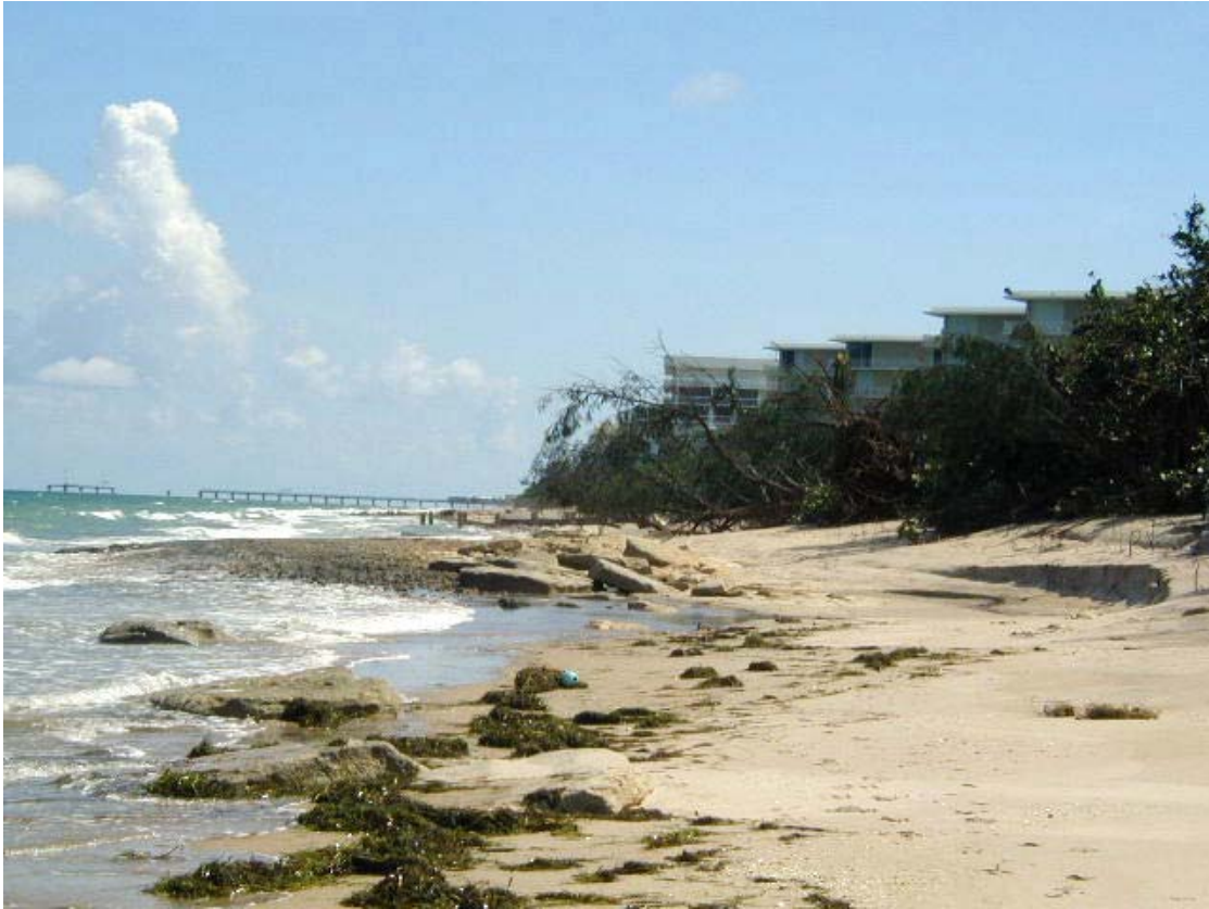
Photo 34. Erosion at Phipps Ocean Park
