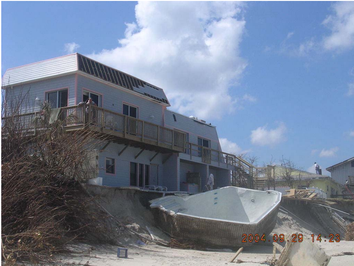
Photo 14: Pool Destroyed (R196)
