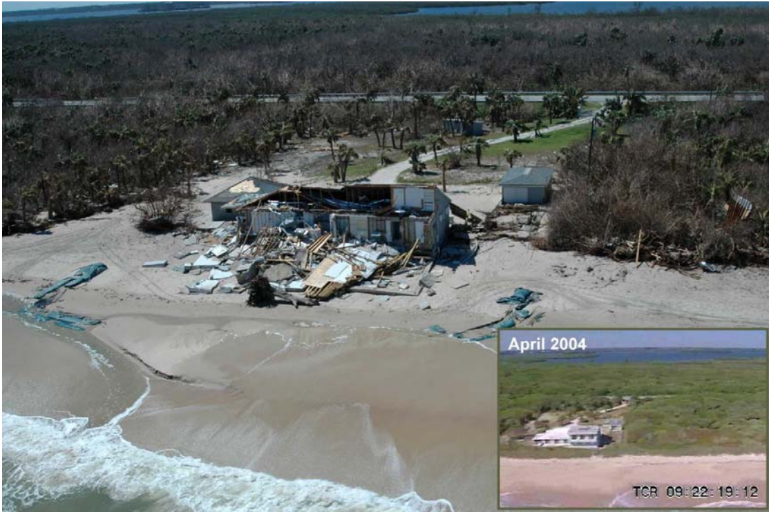
Photo 27: Destroyed Quadraplex, North St. Lucie County (R2)
