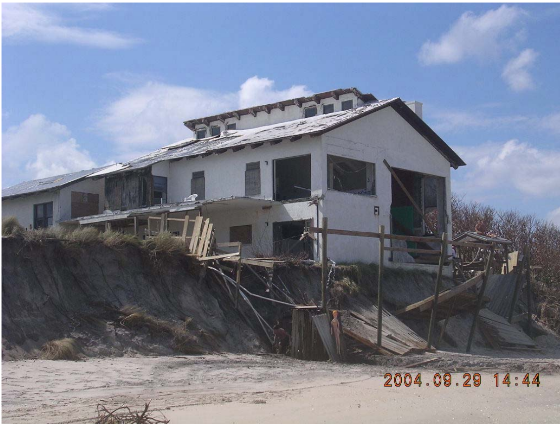
Photo 13: Damage to Residence, Florida Beach
