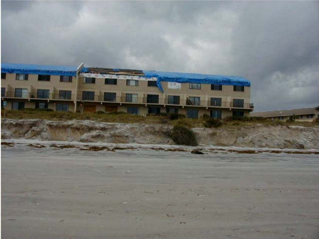
Photo 1: Anastasia Island Erosion at R193
