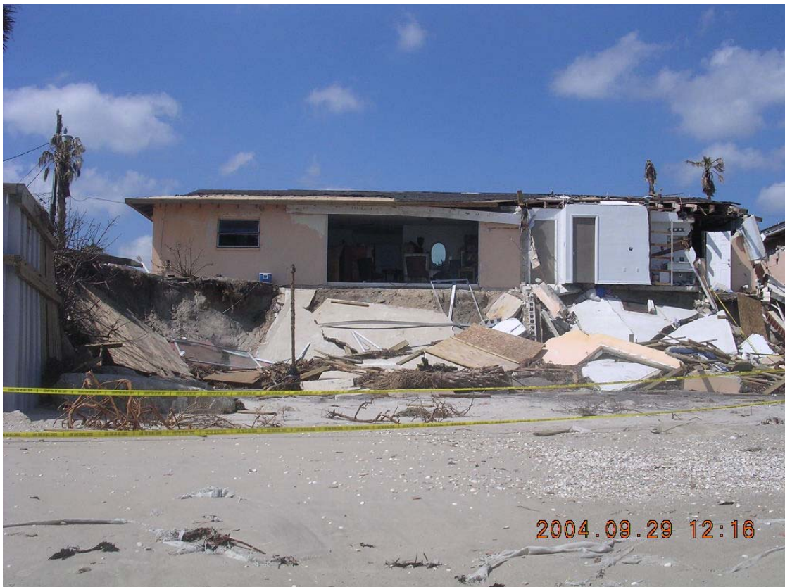
Photo 10: Damage to Residence on Shell Street, Satellite Beach
