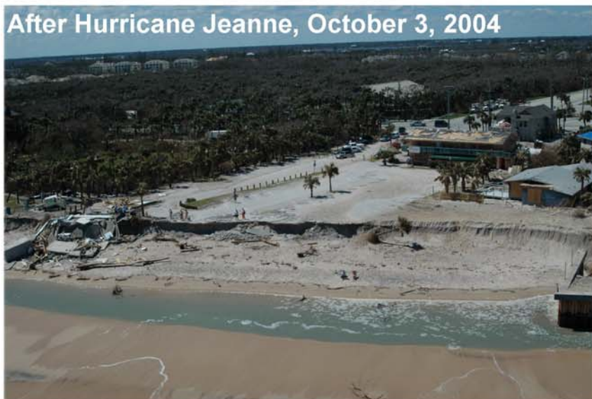
Photo 17: Erosion and Damage , Wabasso Beach Park
